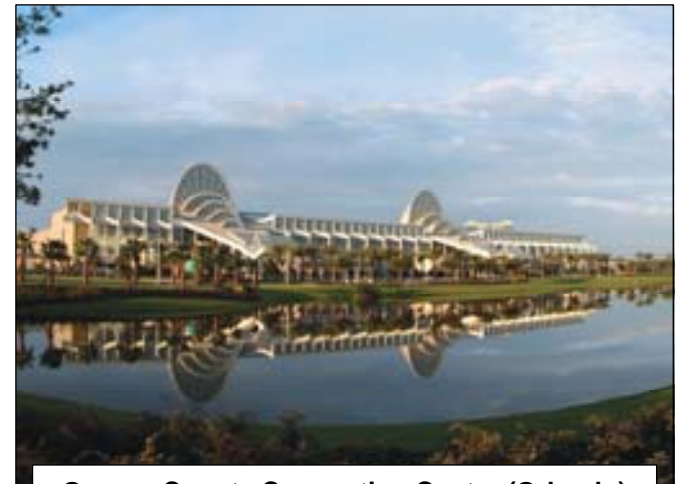
Orange County Convention Center (Orlando)
