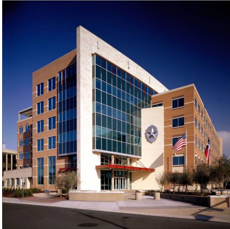
Jack Evans Police Headquarters - a six-story structure is just over 350,000 s.f.
