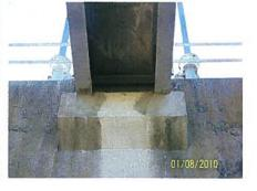
1.1.3 Corps. ID No. 102 – Charlie Pump Station, West Levee – This "M" item noted scaling concrete on the bridge support corbel under the bridge girders at the control structure.
