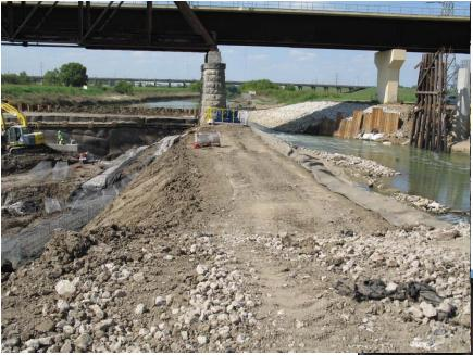
Contractor built a cofferdam and diverted the river channel to be able to work in a dry area
