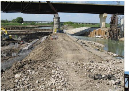
Contractor built a cofferdam and diverted the river channel to be able to work in a dry area
