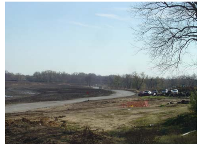
Lower Chain of Wetlands Construction Site
