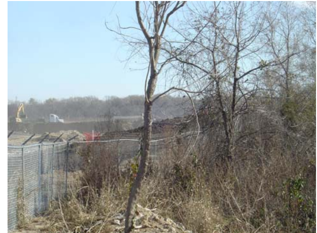
Lower Chain of Wetlands Construction Site
