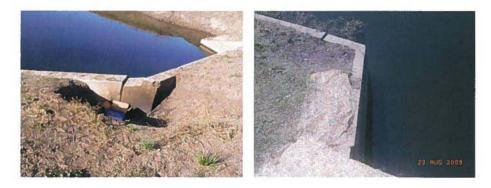
1.2 Corps. ID No. 220 – Rochester Gravity Structure, Rochester Levee – This "U" item indicated Sta. 89+00 had intake gravity flow structure that had depressions on the gabion slopes on both sides of the intake caused by erosion of soil material under the gabions next to the wing walls. The right side had a 2 foot deep gully next to the wing wall (exposed/washing out of bedding) and the left side has a 18'L x 10'W area depression on the gabion slope next to the wing wall.
