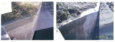
1.4.5 Corps. ID No. 181 – Little Coombs Creek Conduit, West Levee – Service bridge abutment had moderate cracking.
