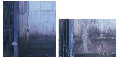
1.4.2 Corps. ID No. 099 – New Baker Pump House, East Levee – Cracking and spalling of the concrete panels at both the right and left side of the trash rack.
