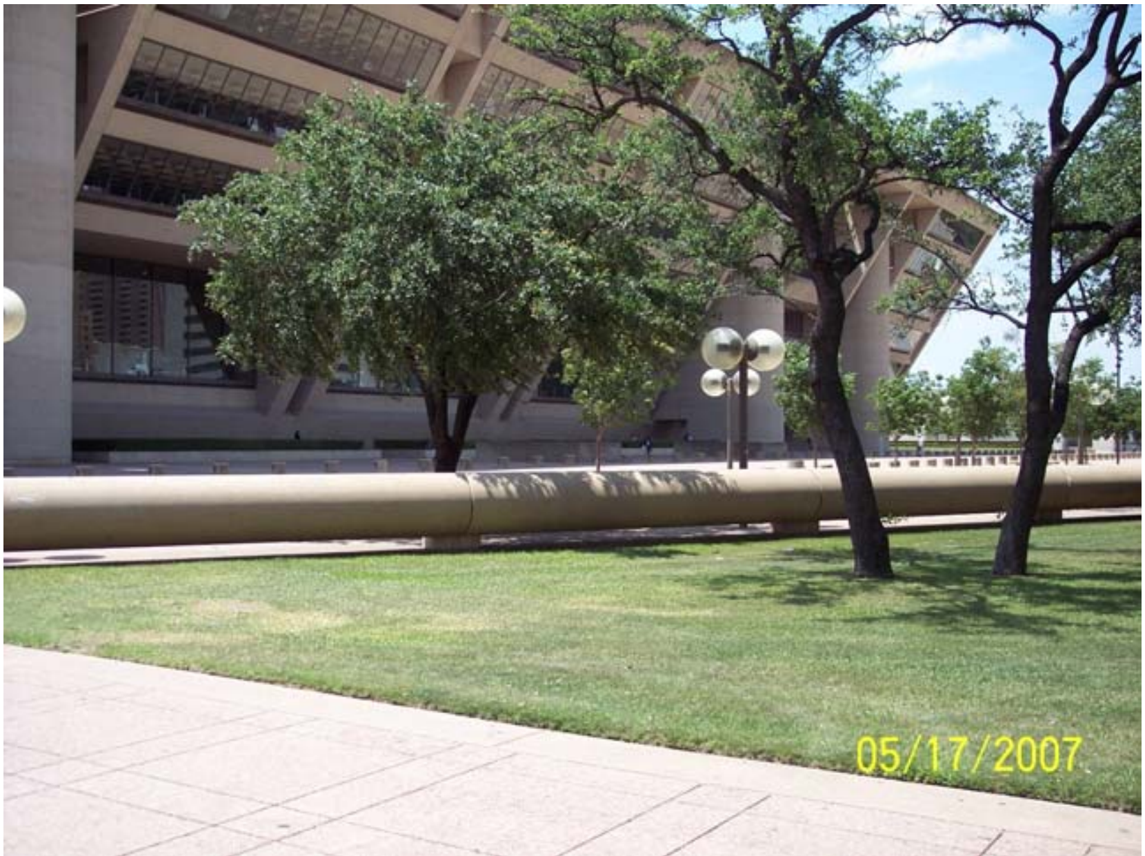
Photo – example of concrete railing on plaza
