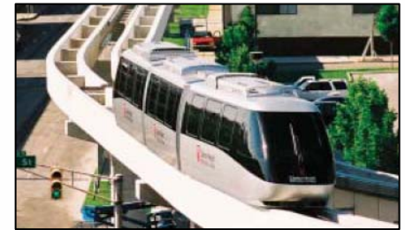
Schwager Davis UniTrak Clarian Health Center, Indianapolis, Indiana
