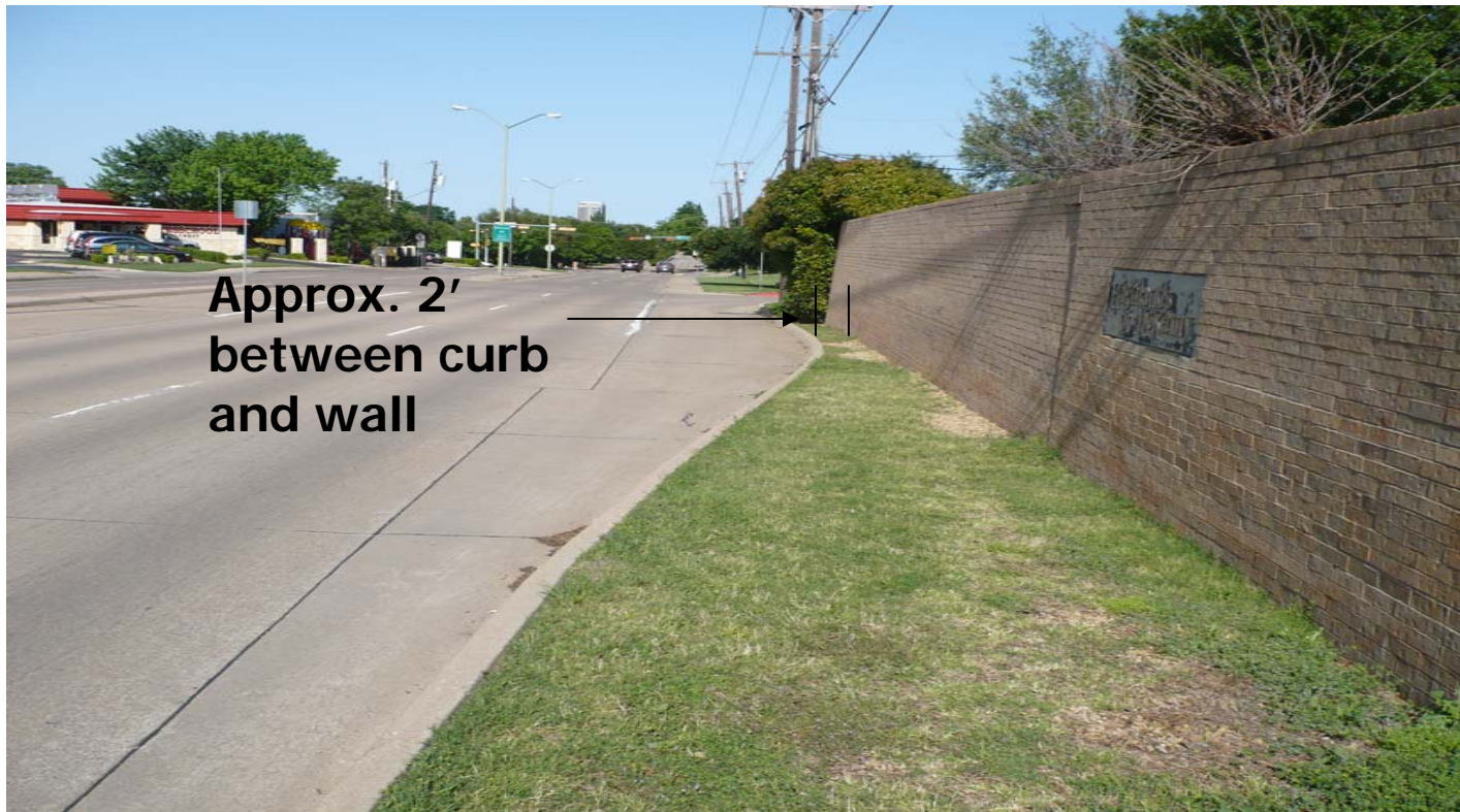
Lack of right-of-way and obstructing screening wall Location: McCallum Blvd.
