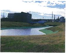
1.2.4 Corps. ID No. 164 – Delta Pump Station, West Levee – Erosion on the right slope (50'W x 80'L x 12'D) of the discharge channel. This item was the same as Corps. ID No. 176 which was addressed in February 2009. The slope was repaired using established levee slide repair procedures.
