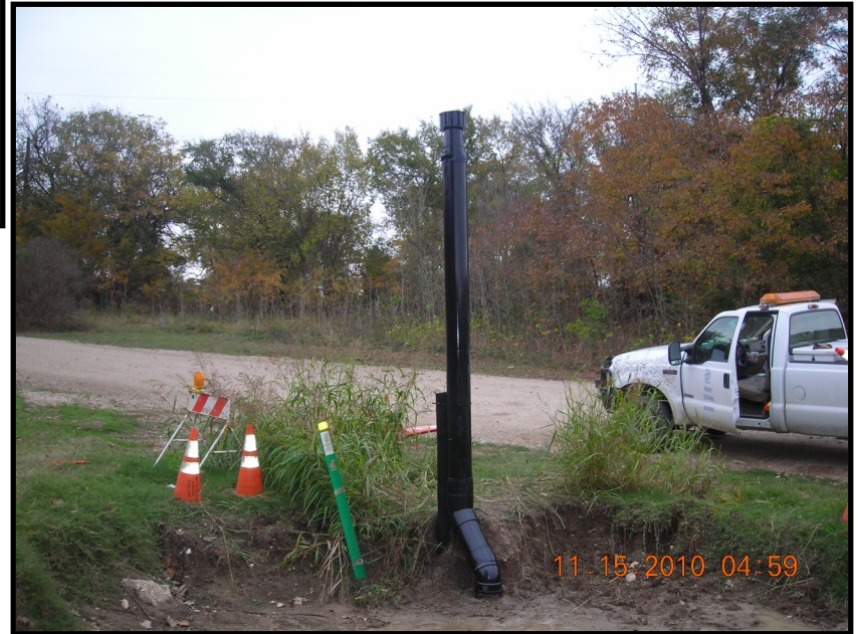
Vent Stack for Wastewater Line
