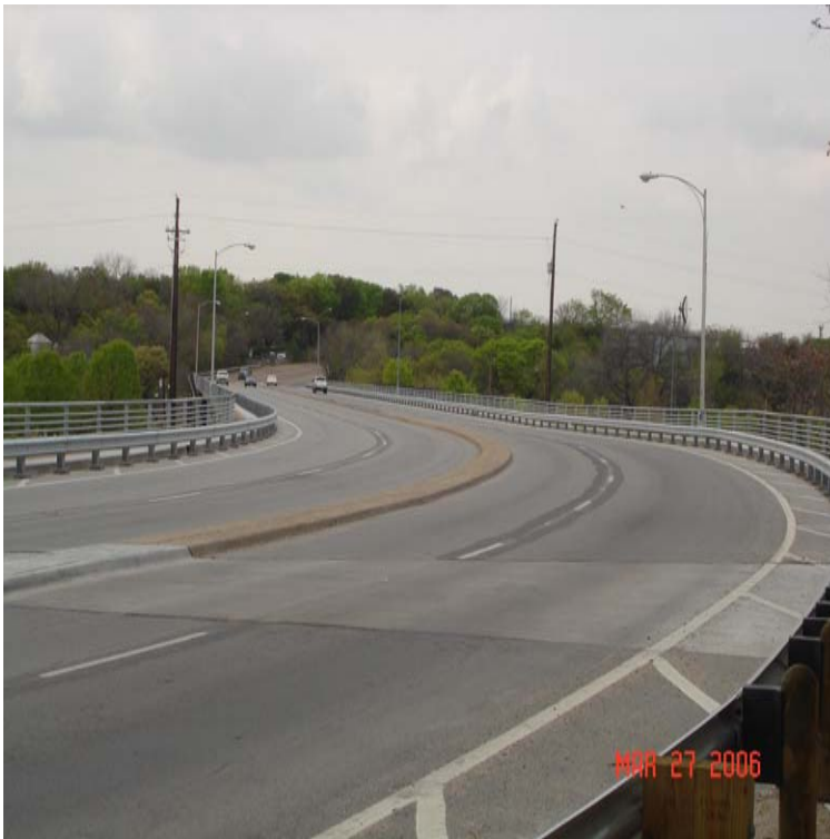
Marsalis Bridge Repairs
