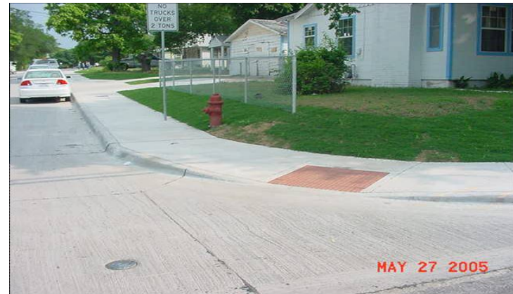
Barrier Free Ramp
