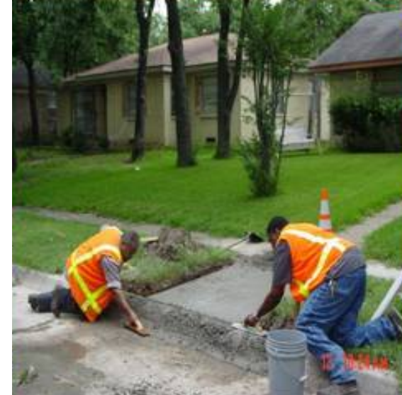
Curb and Gutter w/Sidewalk
