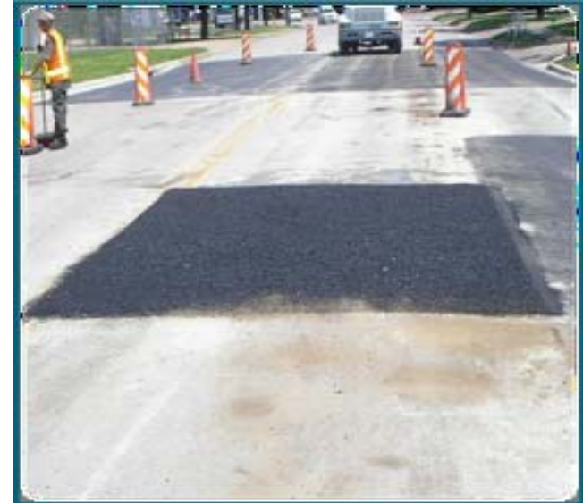
Full-Depth Asphalt Repair
