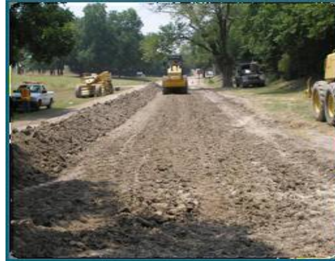
Full-Depth Asphalt Repair
