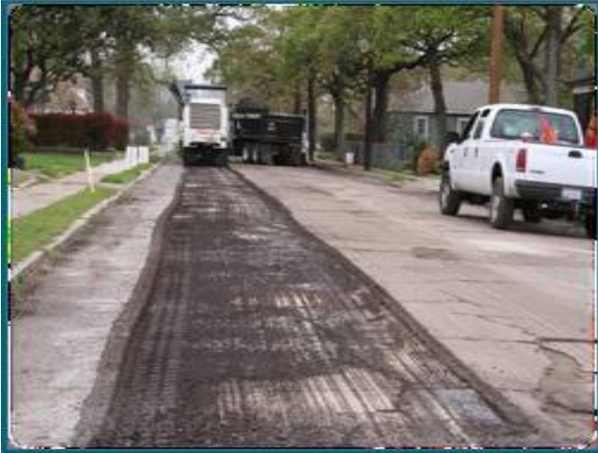
Street Overlay (Rehabilitation/Restoration)
