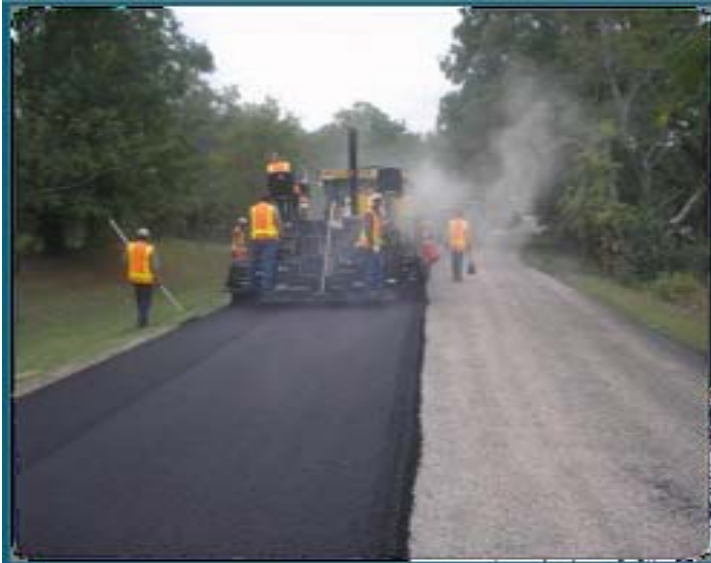
Street Overlay (Rehabilitation/Restoration)
