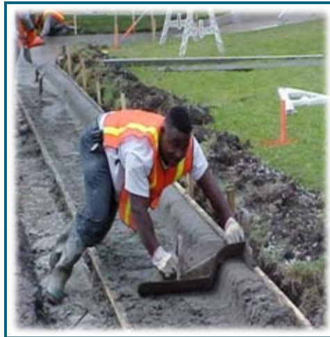
Curb and Gutter
