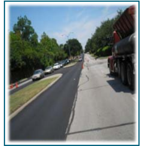
Slurry Seal/Micro Surfacing
