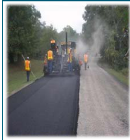
Rehab/Restoration Overlay
