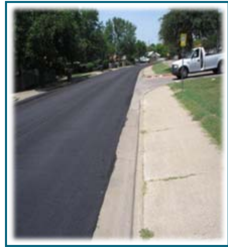
Slurry Seal/Micro Surfacing
