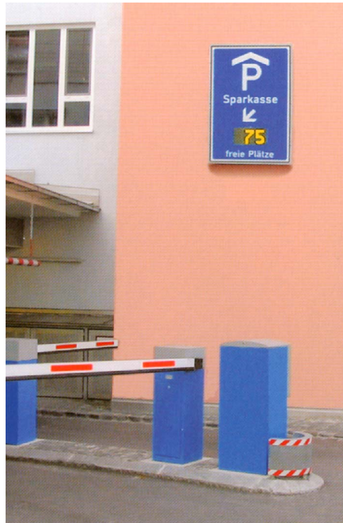
Dynamic sign at car park entrance
