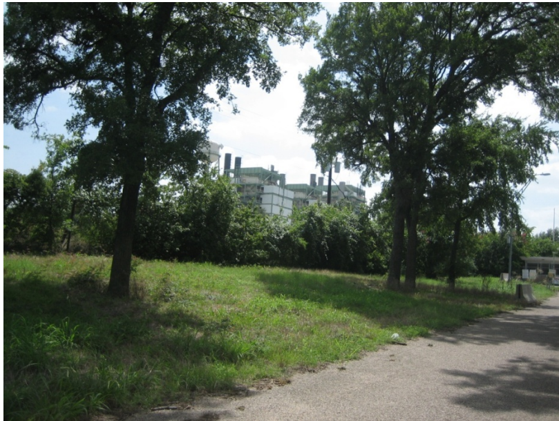
Former power plant.
