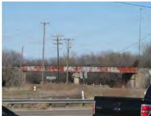
Figure 4.11 (Top) Existing Area 4 Development
