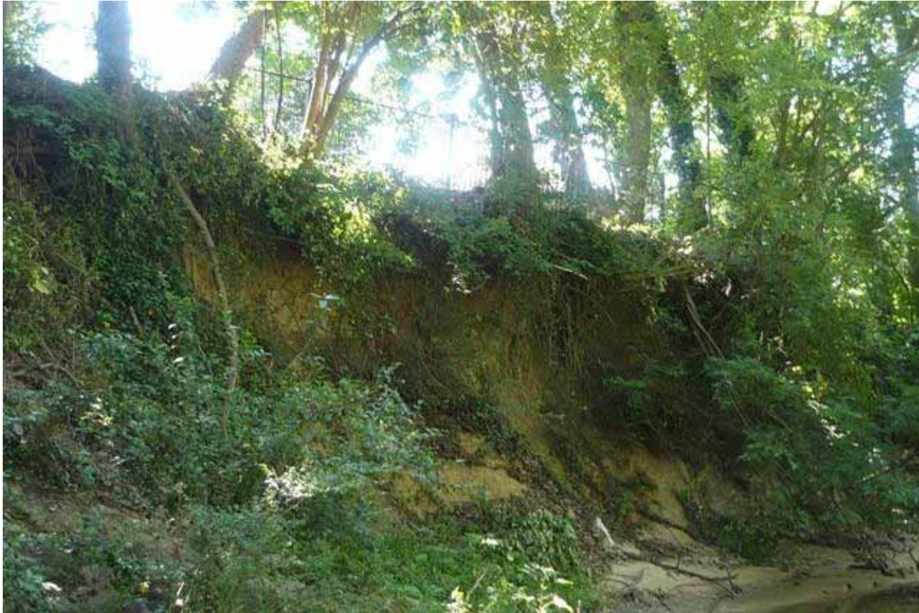
Vertical bank with undercutting present
