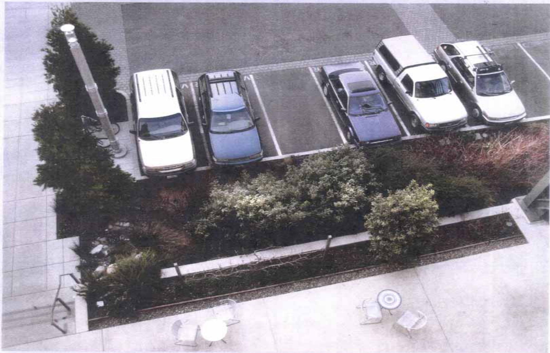
Runoff from parking lot is directed to an infiltration area
