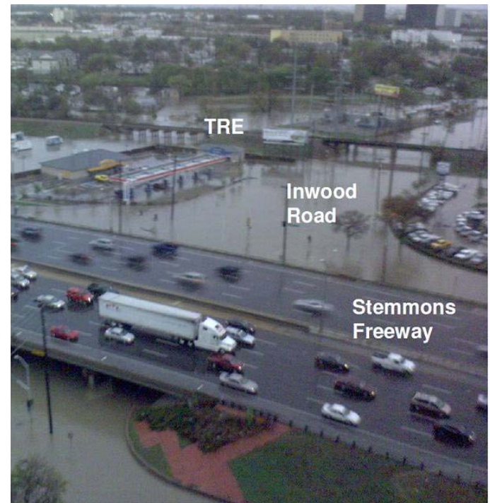
Road at Stemmons Freeway (IH35E), Record Crossing Sump Area - March 19, 2006
