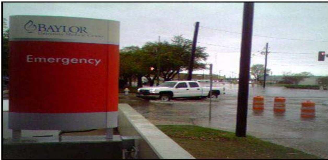
Flooding of part of Baylor Hospital facilities on March 19, 2006
