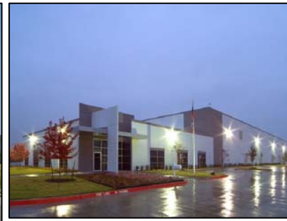
Mountain Creek Business Park
