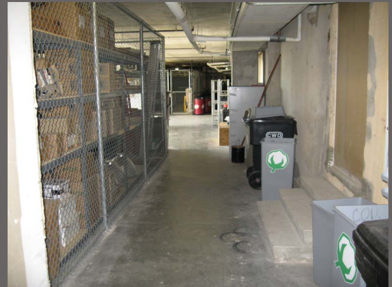
Existing Press Box Level 4
