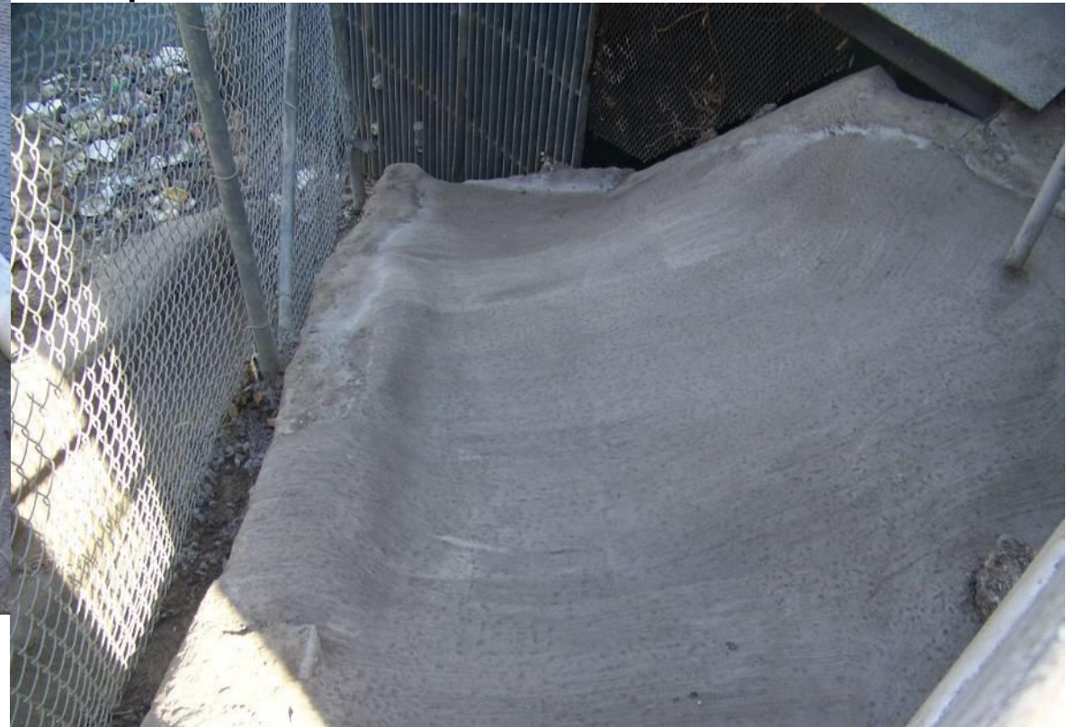
Repaired Concrete Flume – Able Station
