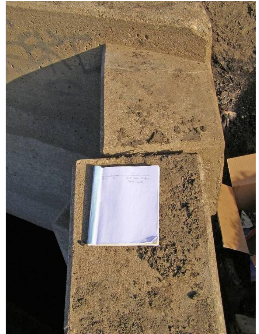
Turtle Creek Pressure Sewer Wall – Separation of Wall 28
