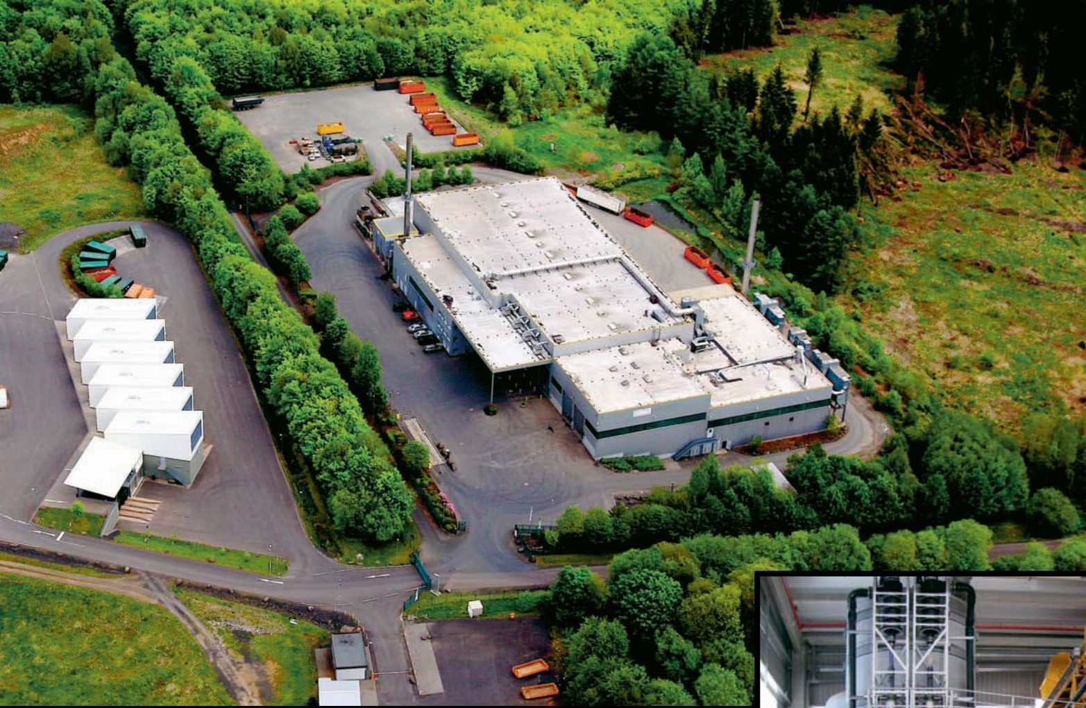
Resource Recovery Facility in Bad Marienberg, Germany
