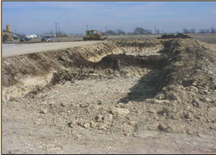
Digging the mud pit
