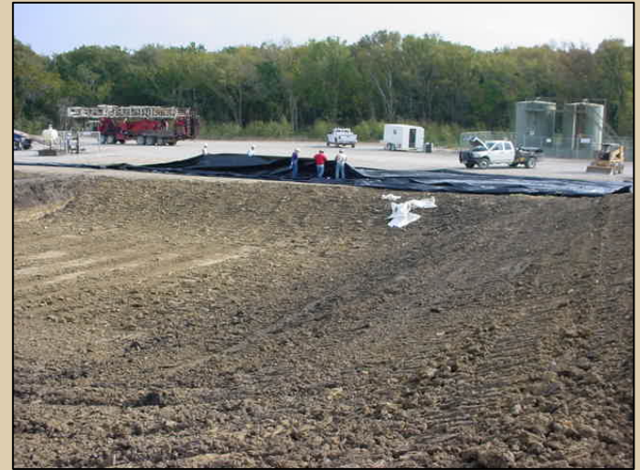
Lining the mud pit
