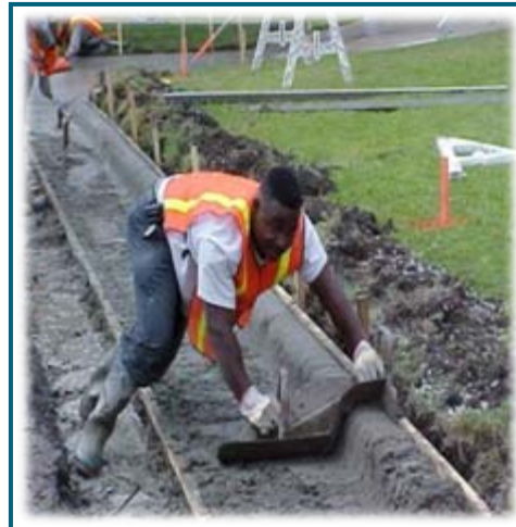
Curb and Gutter
