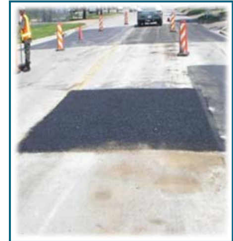
Full-Depth Asphalt Repair
