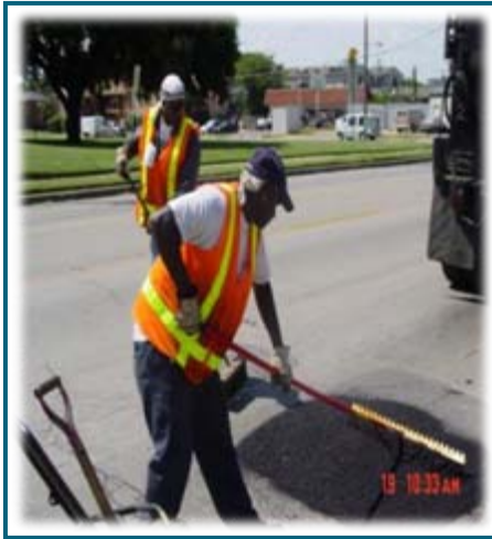
Pothole Repair
