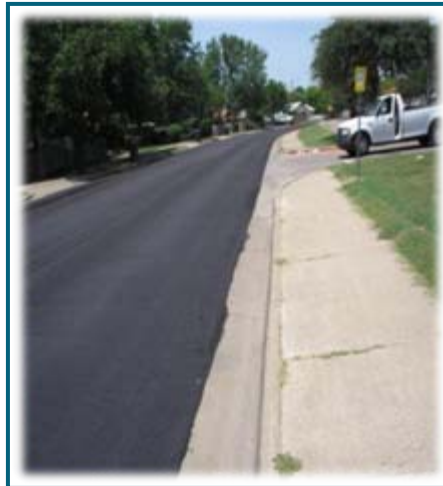
Slurry Seal/Micro Surfacing
