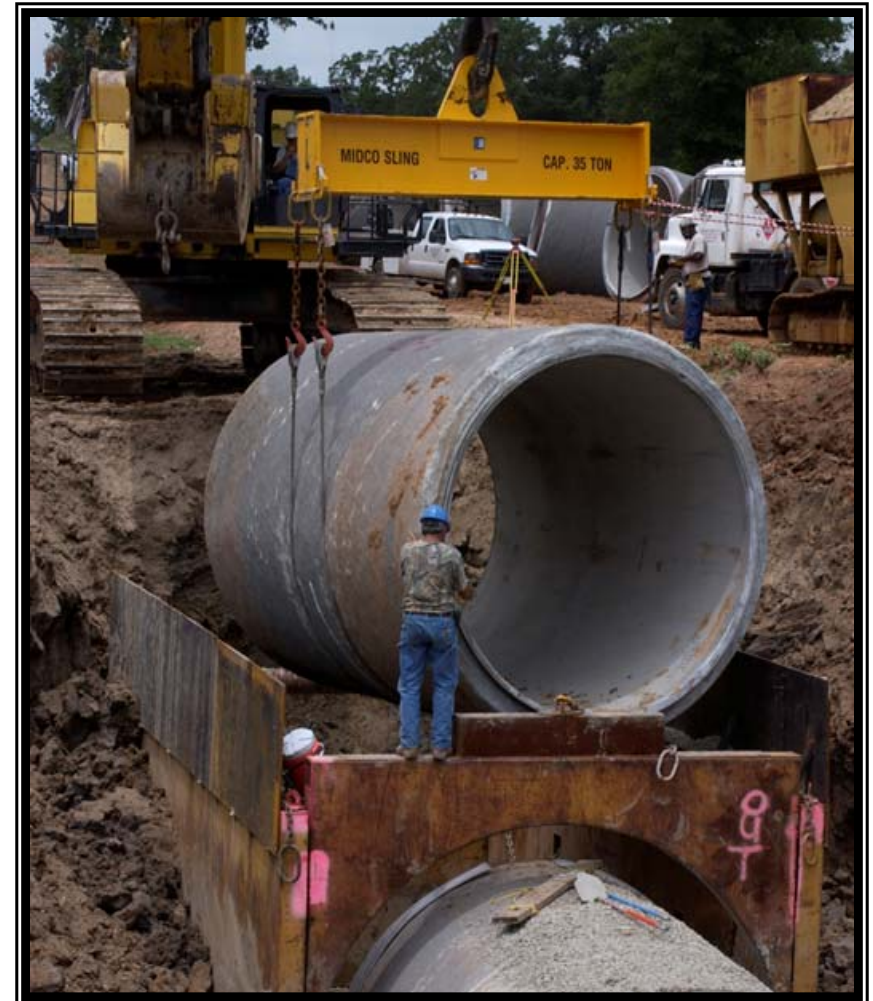
Lake Fork pipeline construction 18
