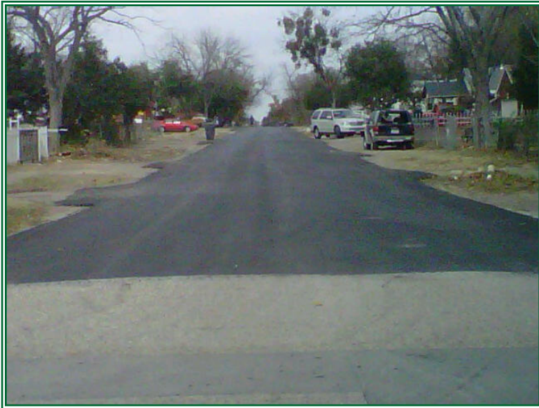
Rehabilitation – Asphalt Street Arizona Ave from McVey to Corning Completed Nov. 2010
